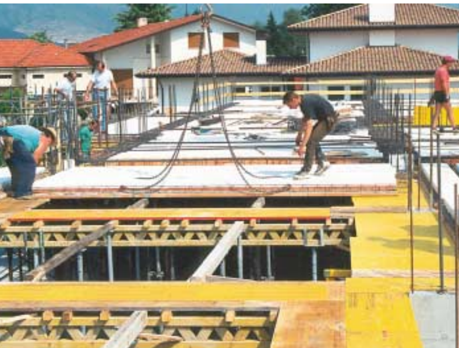
Fig. 13 - Posa in opera dei pannelli. The installation of the panels.
